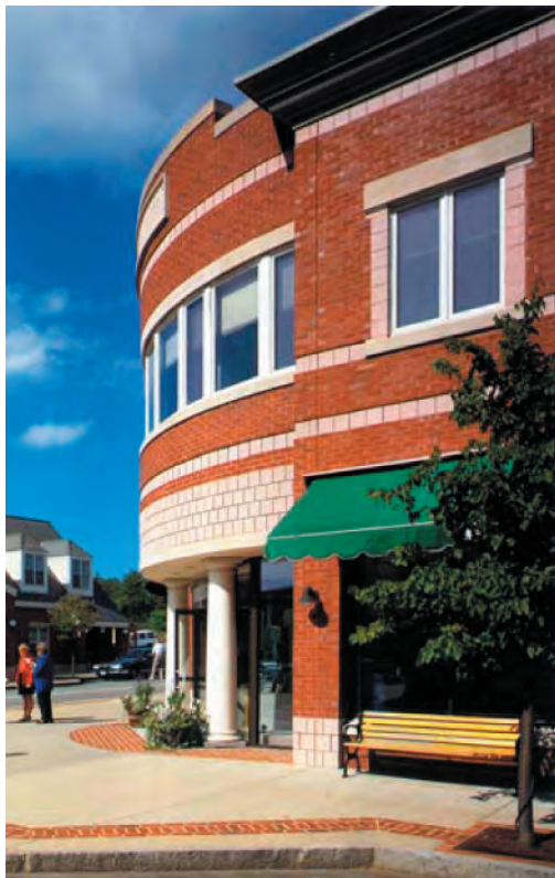
Photo 24: New buildings can compliment without replicating.
