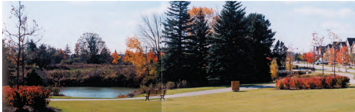
Photo 12: Stormwater Management Facilities as Open Space amenities (Legacy, Markham)
