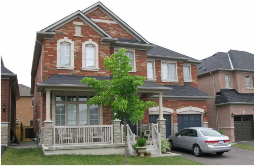
Photo 18: The impact of garages on the streetscape can be minimized by limiting their degree of projection from the main façade of the building.
