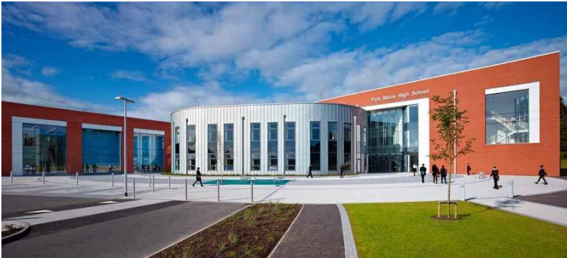
Photo 27: Architectural articulation should reflect the building's landmark status.
