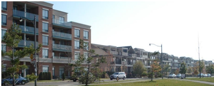
Photo 21: Pairing of medium and high density buildings creates a good transition to adjacent low density areas.
