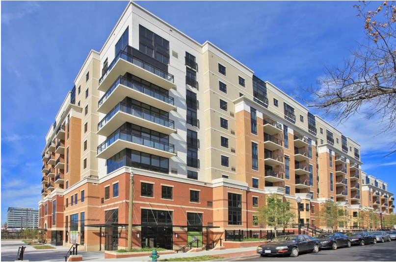
Photo 24: Architectural articulation that enhances the streetscape includes the use of balconies, material differentiation and wall plane changes. Where long street walls like above are created, wall plane changes help break the large massing of the built form.
