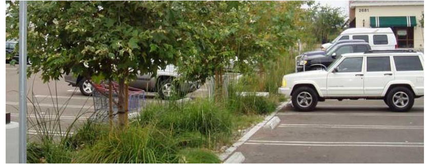
Photo 1: The use of bio-swales in parking lots helps address sustainable development practices.
