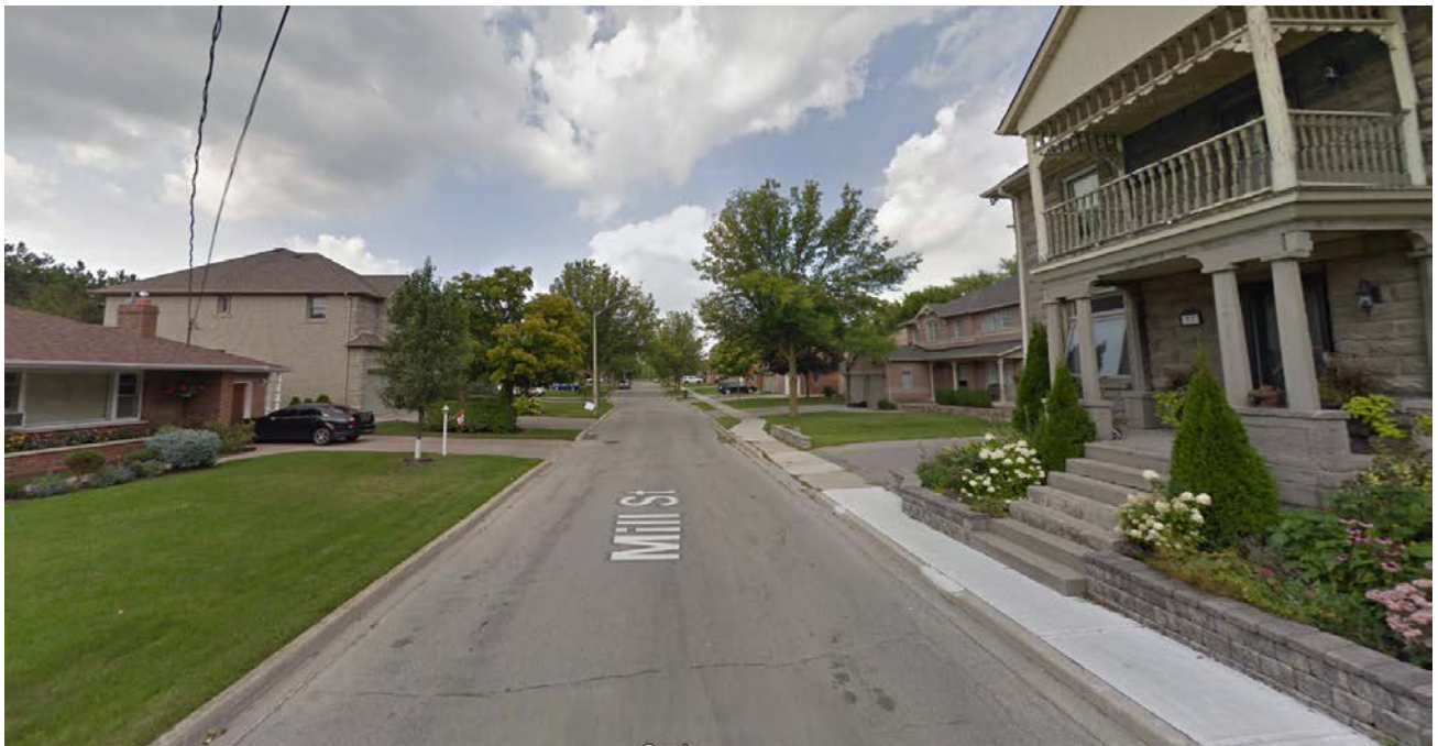
Looking north along Mill Street. The subject property is located on the right (Google Maps, 2018).
