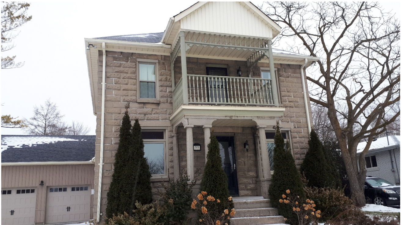
Facing east towards the subject property, with the decorative concrete porch and wooden balcony in view (Parsons, 2019).
