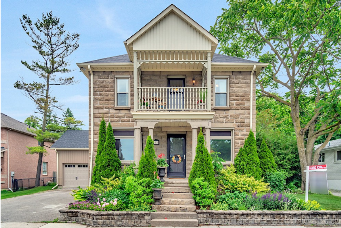
Frontal photograph of the subject property from the recent sale of the property (Trentadue Torres Group, 2019).
