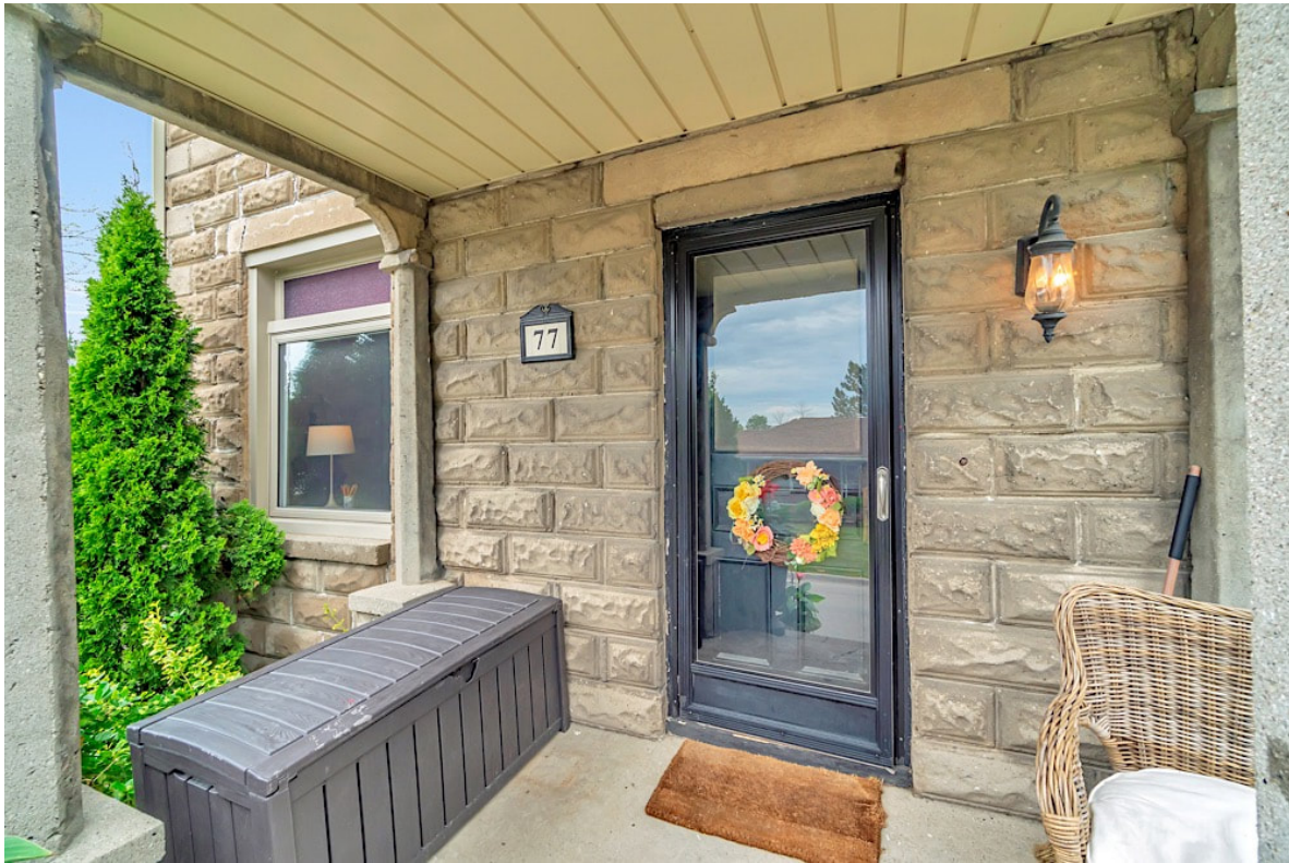
Showing the condition of the front porch with an early or original wooden door, concrete columns, and a close-up of the rusticated concrete block intended to emulate the exposed aggregate facing of stone (Trentadue Torres Group, 2019).
