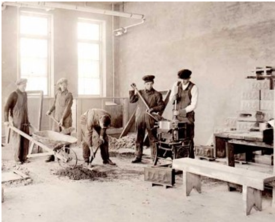
It is very likely that the blocks were produced at the North American Cement Block & Tile Company in nearby Gormley, which was in operation prior to the construction of the subject dwelling (Classic Rock Face Block, Gormley Heritage Conservation District Inventory).
