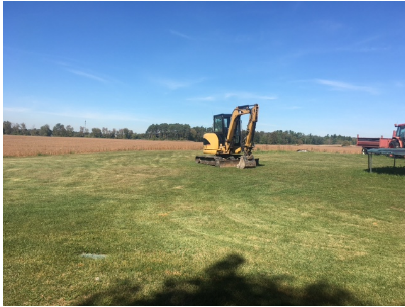
Plate 9 Shows conditions for test pitting.
