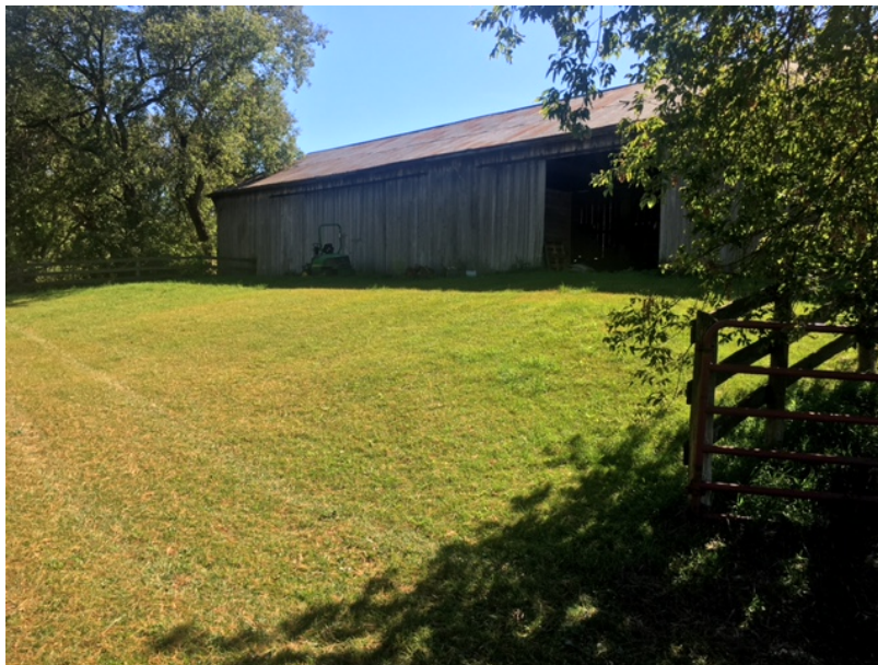
Plate 14 Shows conditions for test pitting and existing structure.
