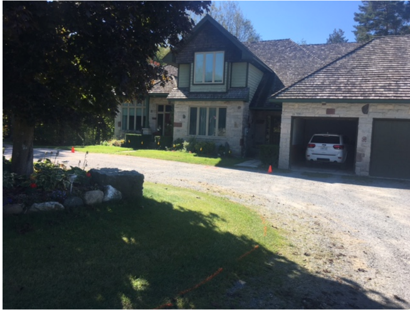
Plate 11 Shows existing structure.
