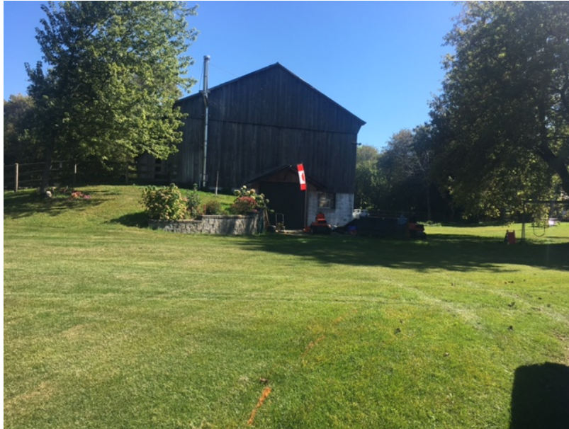
Plate 13 Shows conditions for test pitting and existing structure.
