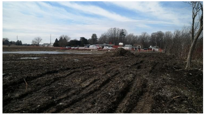
Photo 4. View along the northern fencerow facing Woodbine Avenue. Pooled water shows where the wetland was previously located (April 6, 2022).
