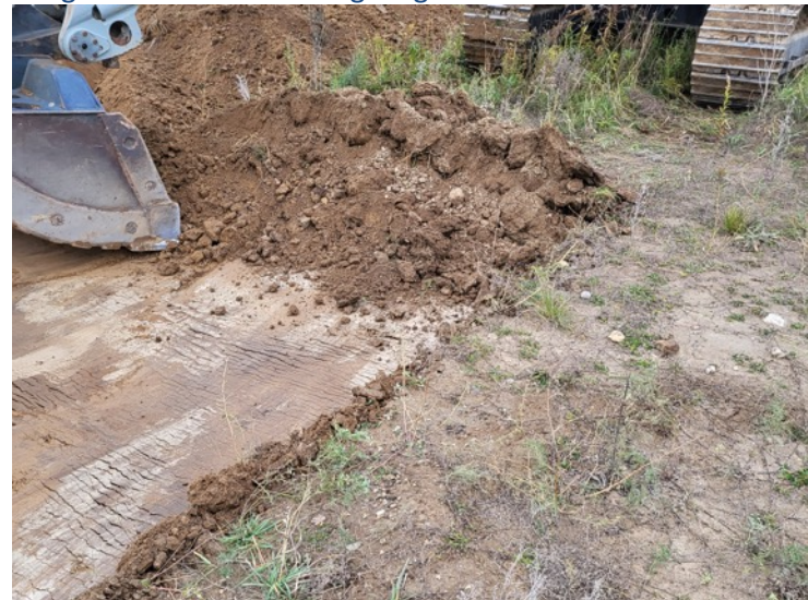
Image 8: Exposure of clay fill underlying thin, gravelly topsoil in the eastern part of the site.
