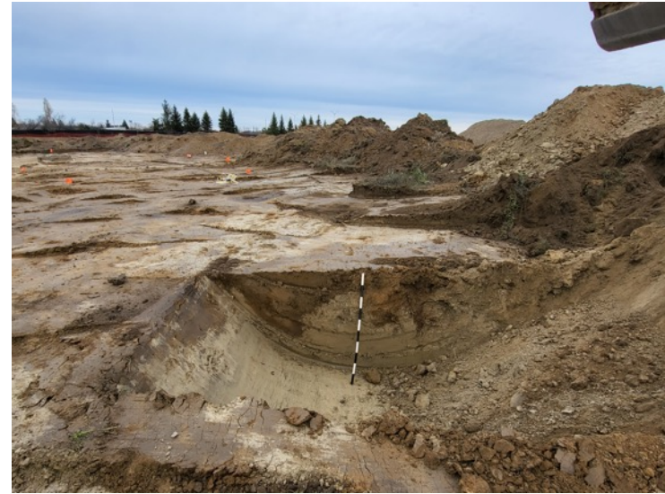
Image 10: Exposure of deep clay fill underlying topsoil in the southeastern part of the site, indicating previous disturbance.
