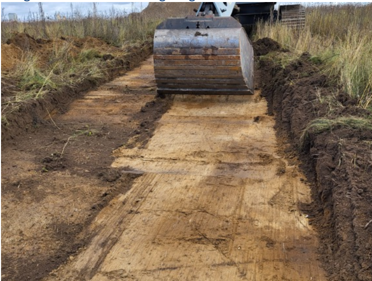
Image 7: Commencement of topsoil removal at the northwest corner of the site.
