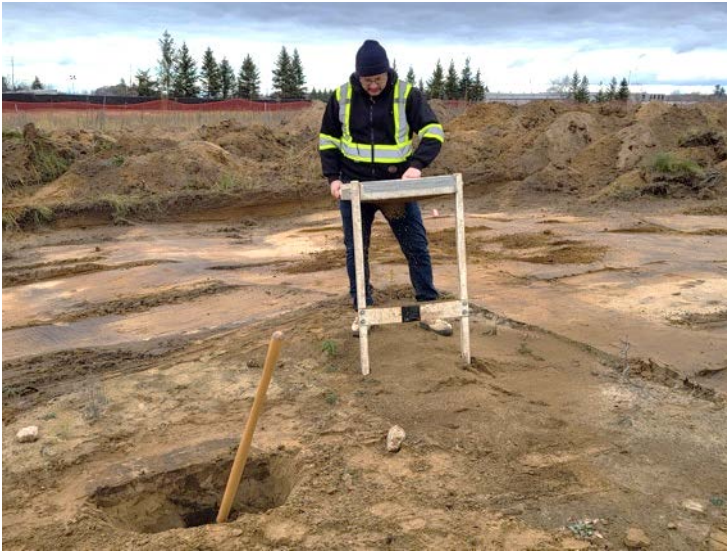
Image 13: Excavation of Feature 1 in progress.
