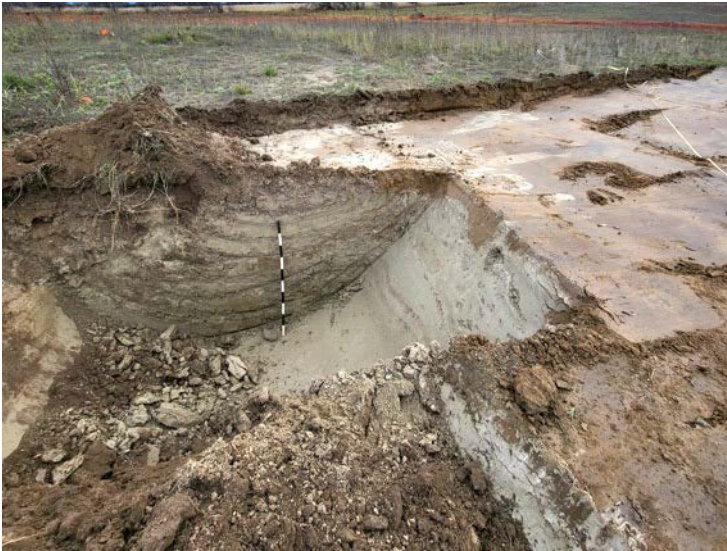
Image 9: Exposure of deep clay fill underlying thin gravel/sand topsoil in the eastern part of the site
