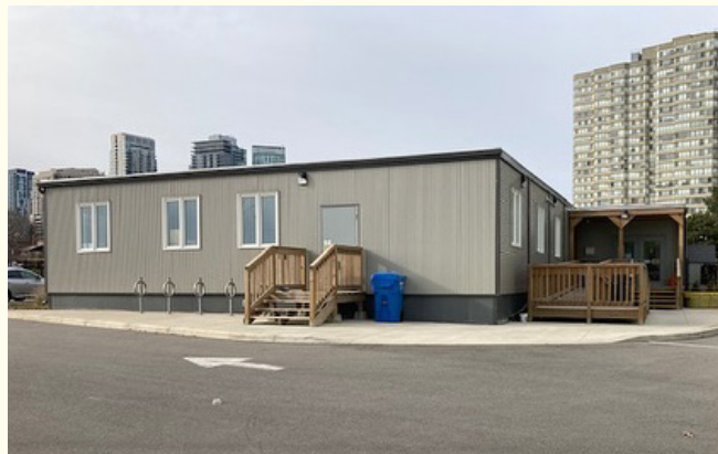
ABOVE: The modular daycare facility that will be relocating to Stouffville.
