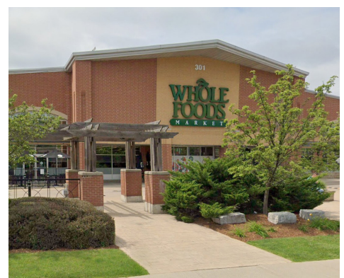
Neighbourhood Retail: Standalone Commercial Building
