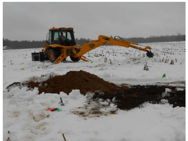
Photograph 6. Test Pit program conducted in Jan 2017 at the Phase Two Property.
